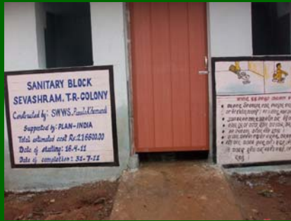
A toilet block at one of the school in Chilika Project
